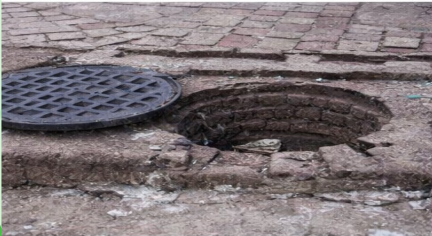
Manholes in Indus valley drainage systems for periodic desilting
