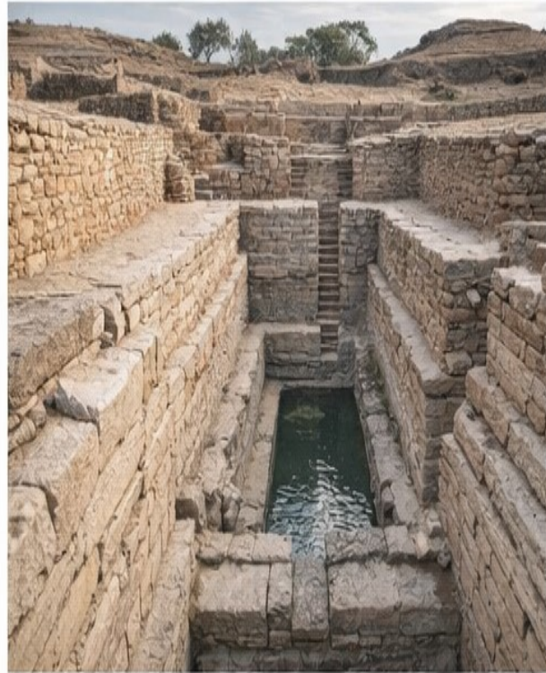
Stepwells store rainwater for year-round supply (Patan, Gujarat)
